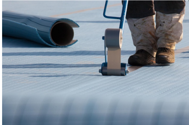
Image 6: Usage of a special tape roller for more efficiency
