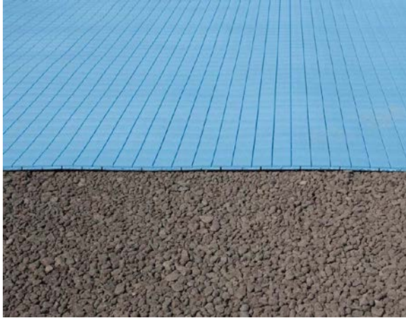
Image 1: Alveosport laid directly on smooth levelled sub-base
