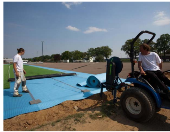
Image 10: using a winch
