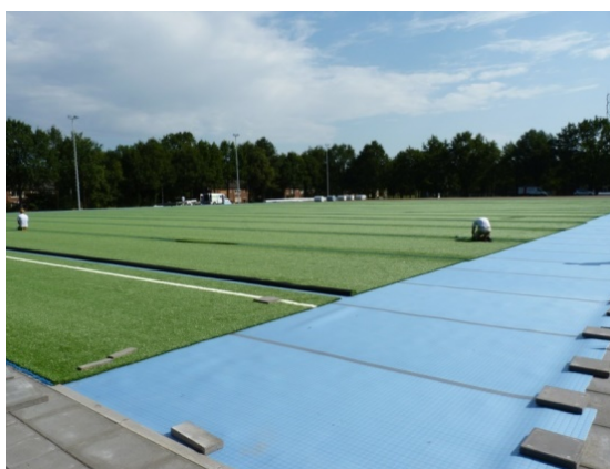
Image 4: load on the side of shock pad and carpet to protect from wind
