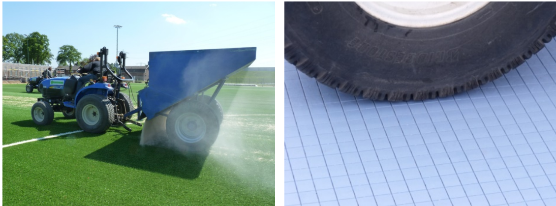
Image 13 & 14: Installation equipment on Alveosport during installation
